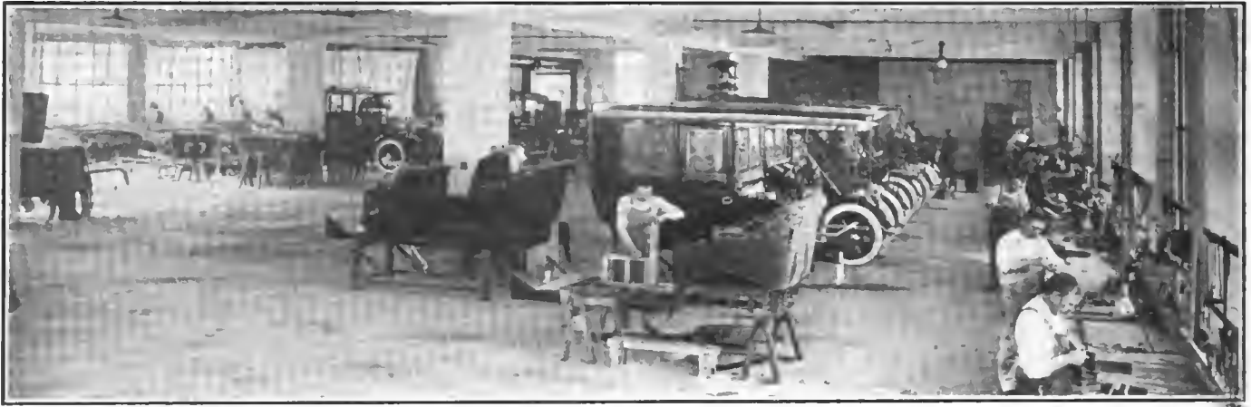
Fig. 1—A portion of the coach department in the new Packard service station in Long Island City
